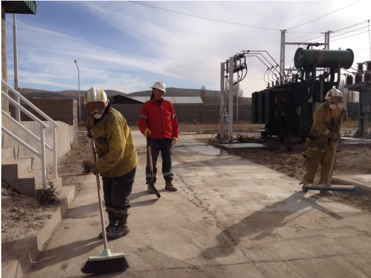
Figure 4 Workers clear ash from a substation in Junin de los Andes, Argentina. This town received ~20 mm basaltic andesite ashfall from the 2015 eruption of Calbuco volcano, Chile, 200 km away (photo credit: Bomberos Voluntarios de Junin de los Andes, Argentina)
